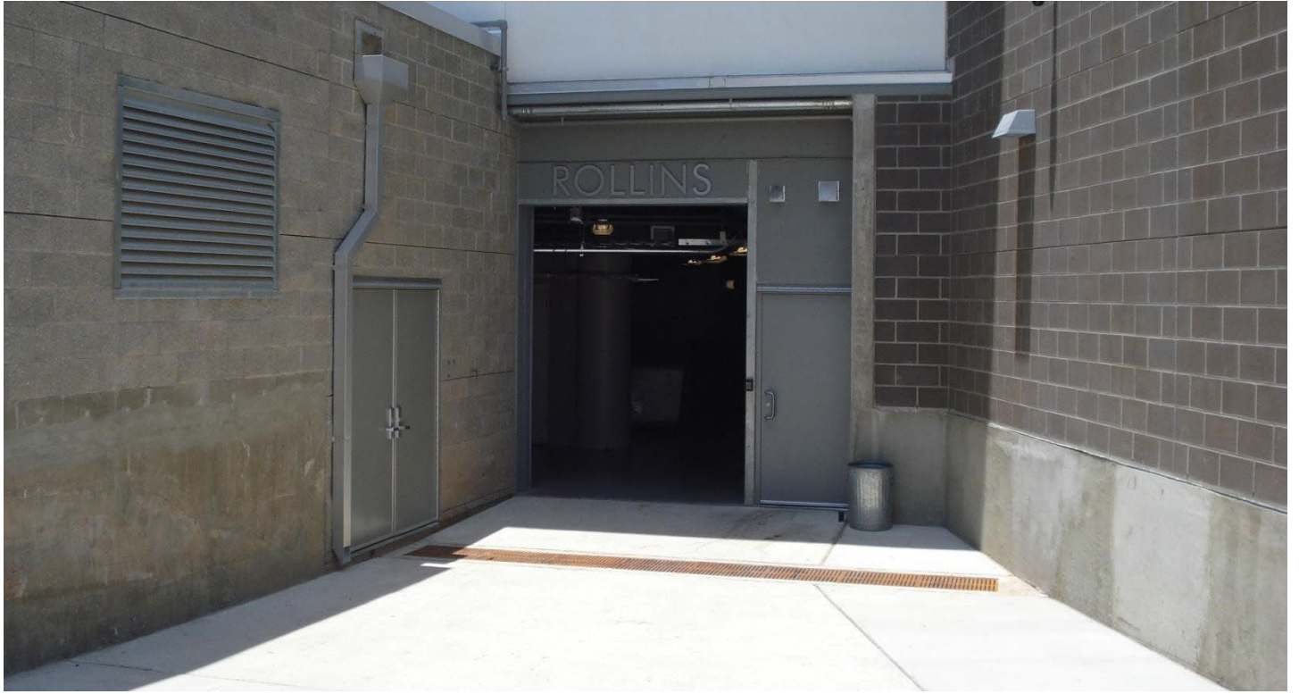
Rollins Studio Theatre Loading Dock
